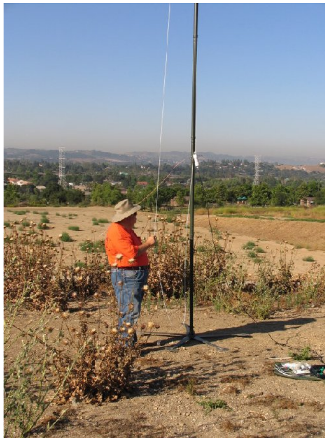
Hoist the antenna slowly! Have helpers at both ends of antenna!
