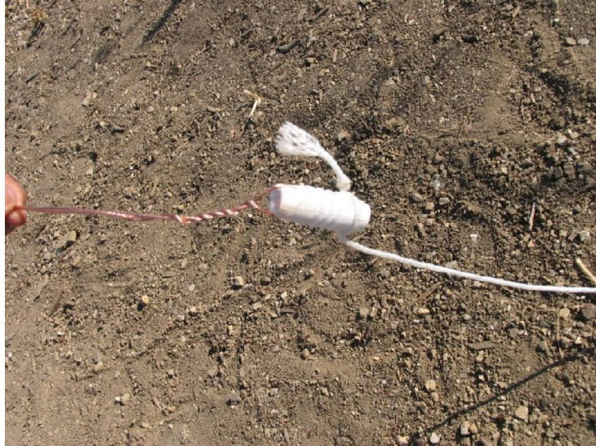
Attach guy lines to dipole insulators
