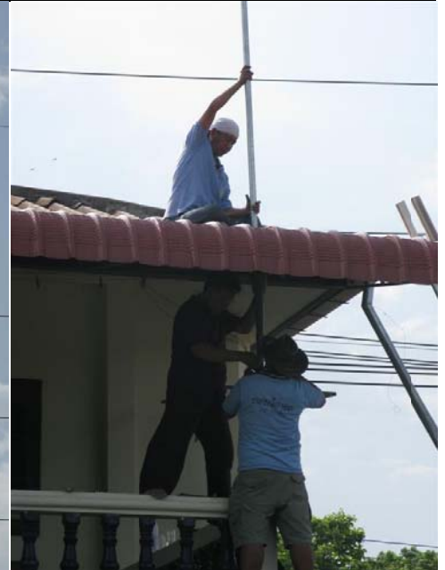
At (above) with AI and Kasem (below) raising the steel mast to set the Isopole to its final height.
