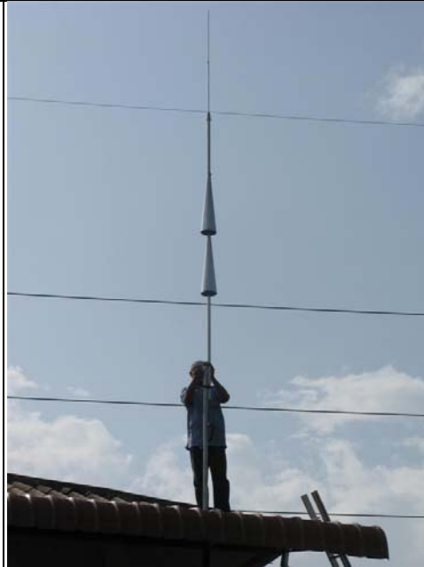
At mounting the Isopole to the steel mast and adjusting the air choke and coax feed line
