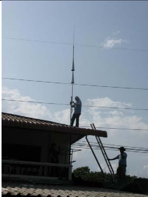
At (HS5PTC) and Kasem (HS5ASA) setting up the Spectral Isopole VHF antenna with E20NXT standing by to assist.
