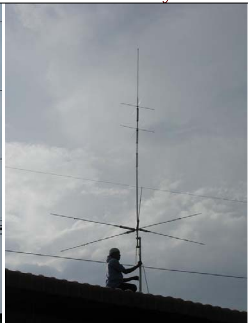
At checks the radials and coax.
