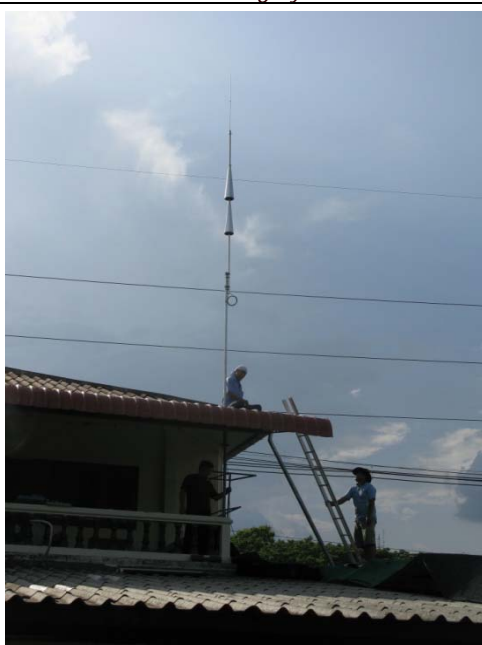
The Isopole feed point is ~8.3 m above ground level.
