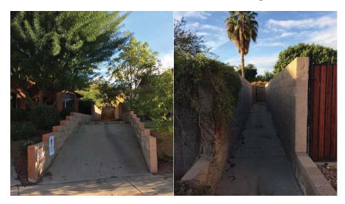
Photo 2 – Concrete Outfall Channels
