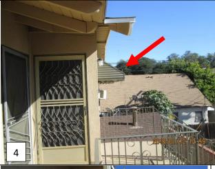
Photo 4 shows the antenna bracket blends into the background. It is barely noticeable with the background clutter of the trees and utility lines.
