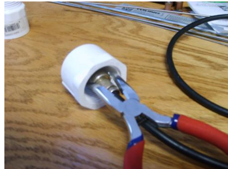
Tighten PL 259 with a needle nose pliers
