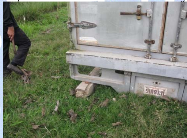
The container is stabilized on stumps and salvaged concrete posts over the uneven ground.
