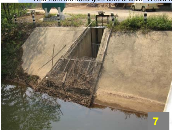
Debris screen at the emergency by-pass flood gate.
