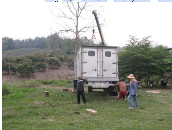
The container is aligned to previously surveyed markers.
