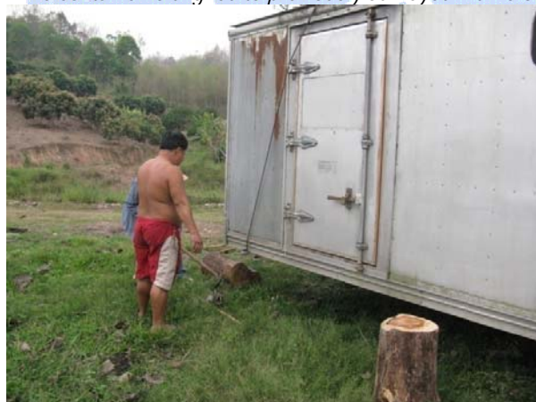
The container is stabilized on stumps and salvaged concrete posts over the uneven ground.
