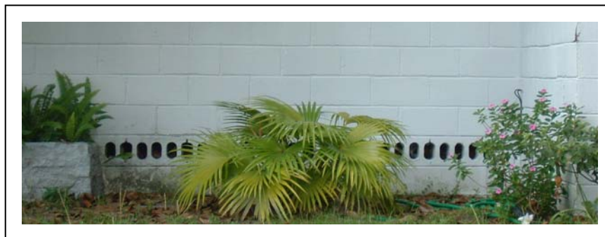
Figure 3-23: Foundation vents (concrete block placed sideways)
