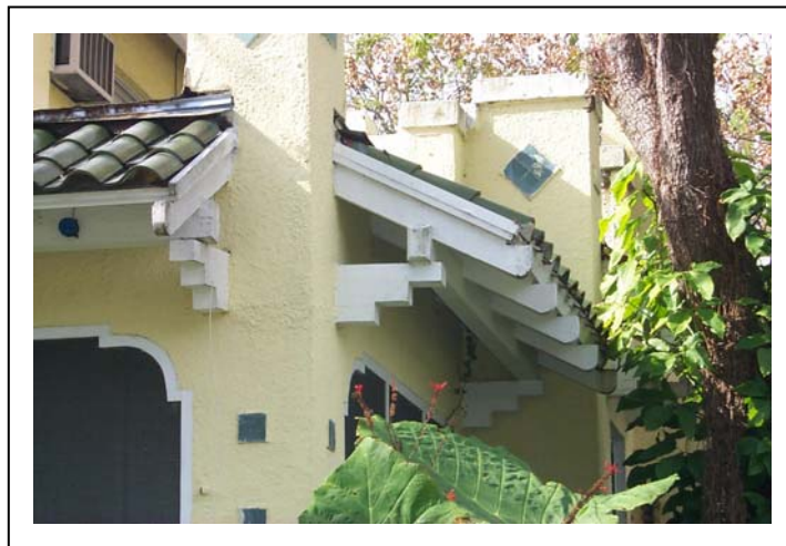
Figure 5-29: Rafter ends
