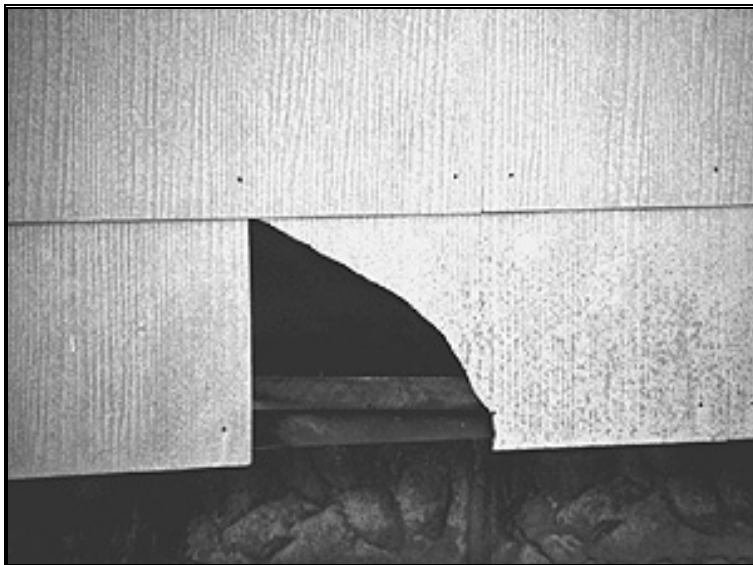
Figure A-1: Asbestos Deterioration
