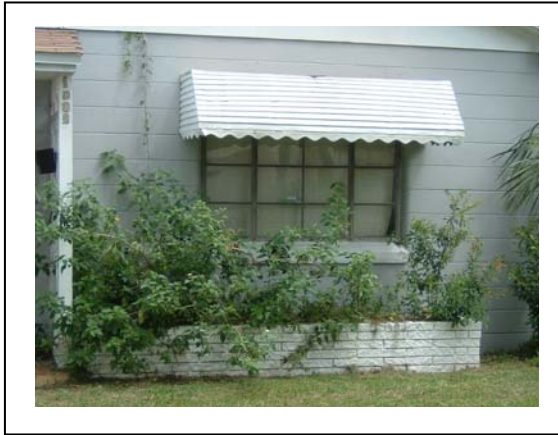
Figure 3-19: Awning, planter, steel casement window
