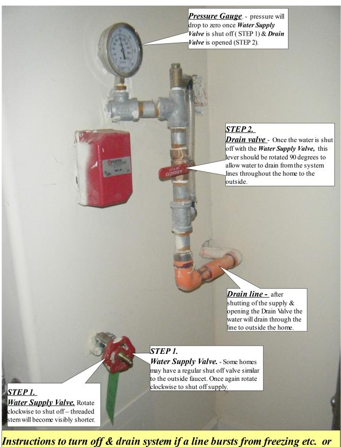
Instructions to turn off & drain system if a line bursts from freezing etc. or after a fire is extinguished by a sprinkler head operating.
