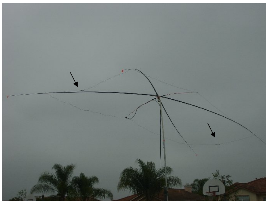
This is a two element beam. Arrows point to insulators that separate the elements
