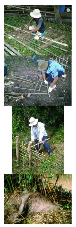
A small check dam is an important water and soil conservation tool. ESSI RTC Staff learned to make, site, install, and maintain simple check dams.
