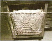
Poor filter maintenance or unfiltered return air will contaminate a condensing coil making it difficult for equipment to function. This unit will require a professional cleaning costing hundreds of dollars. In the long run proper filter maintenance is cheaper!
