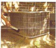
so that it can pull in plenty of fresh air. Coil blockage increases operating cost and shortens equipment life cycle.
